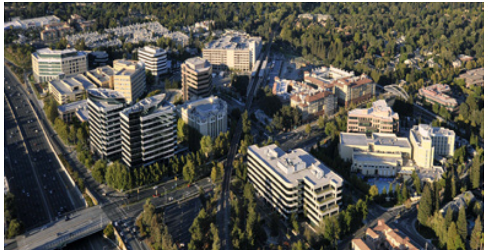
An aerial view of Contra Costa Centre
